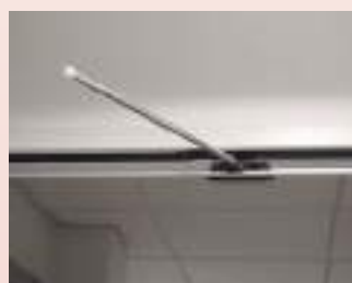
Closing regulator on double leaf door (standard)
