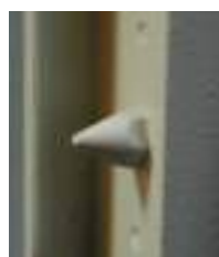
Bolts fire rated Bolts on leaf and strikes in the frame
